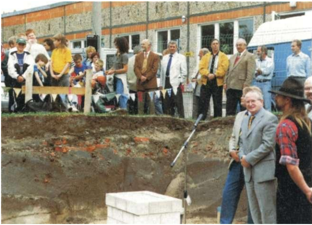
Erster Spatenstich Therapiehalle 1998 The first sod is turned at the therapy hall, 1998
